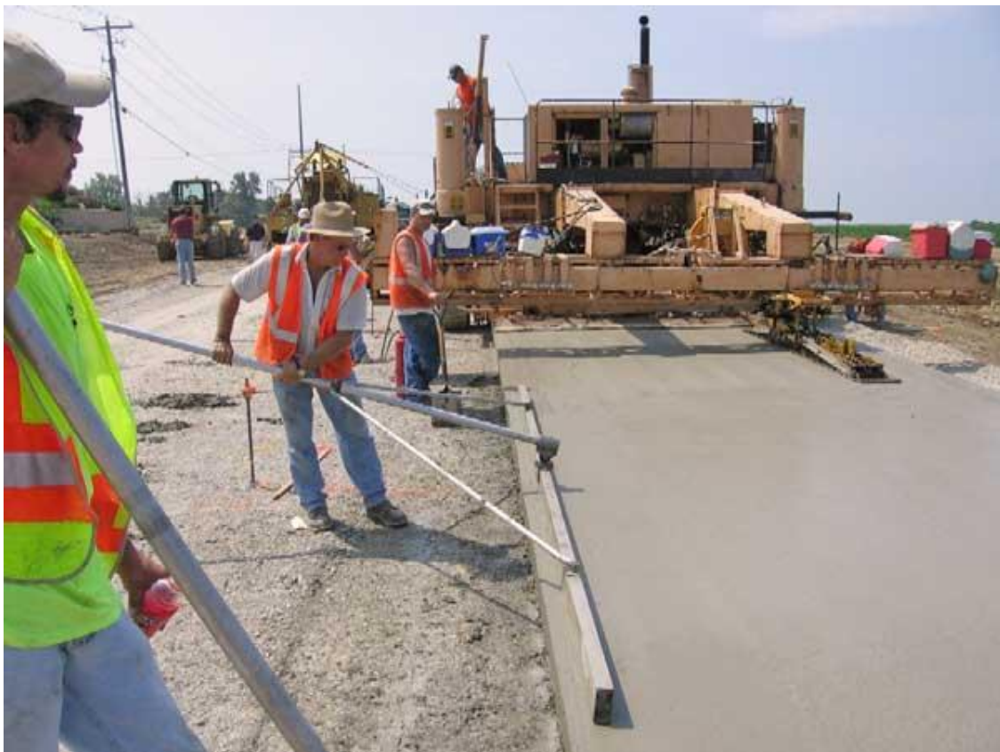
Figure 2.2: Concrete road under construction
